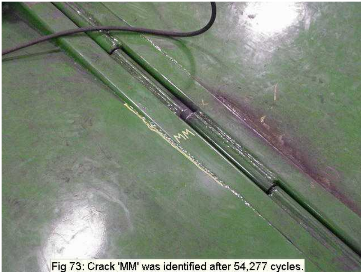
Figure 6 – Failure on Top Deck of Centre Cutter
