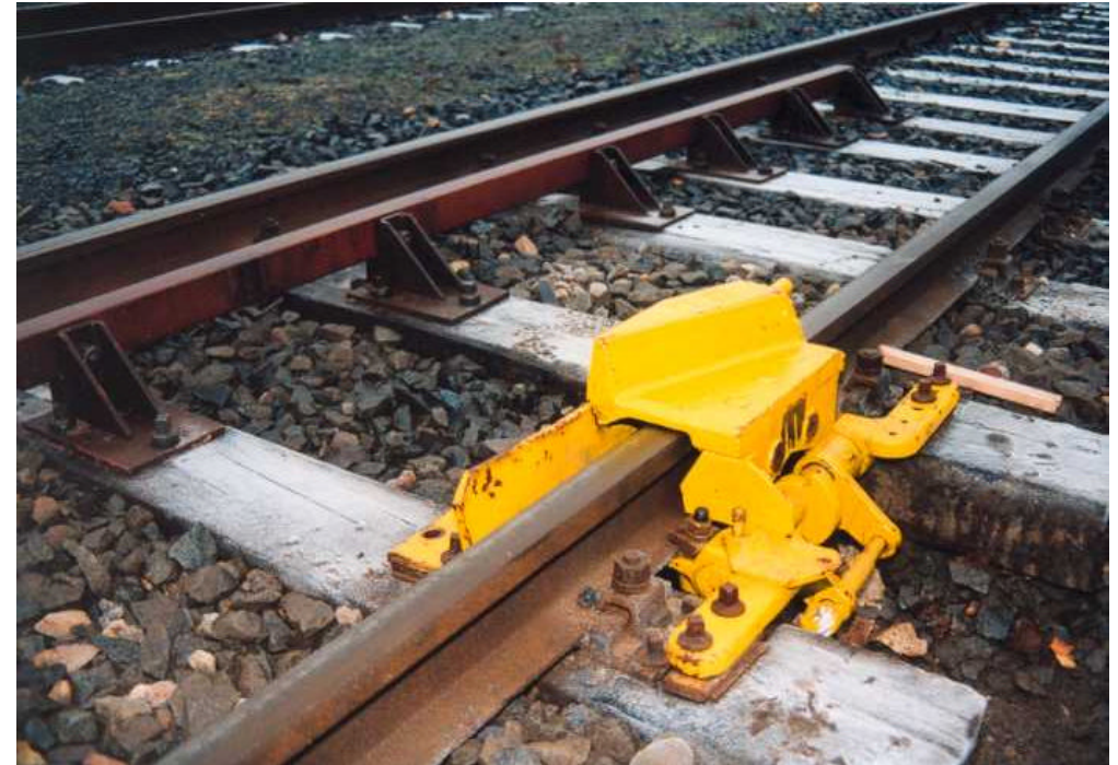
Derailer and guard rail
