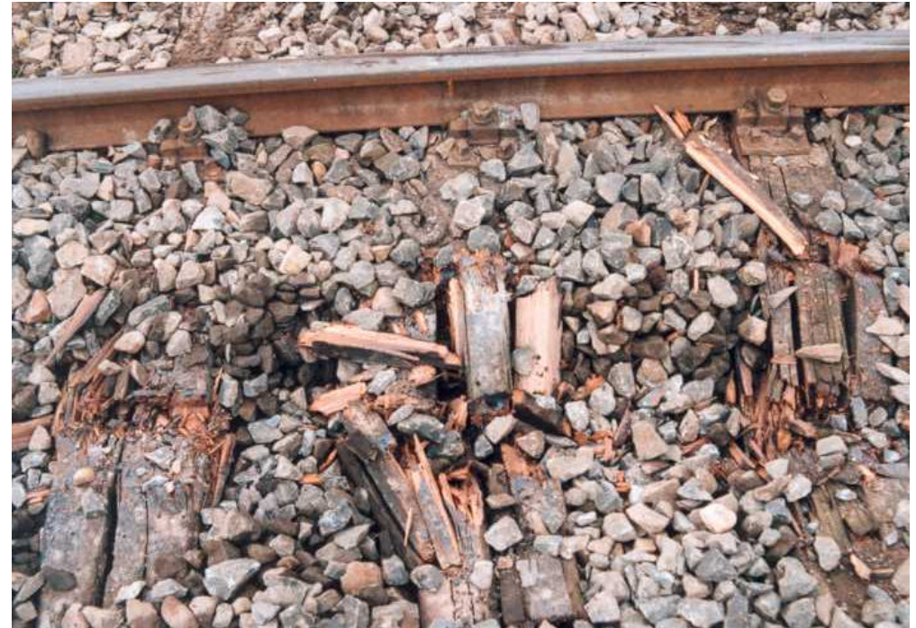
Damaged sleepers
